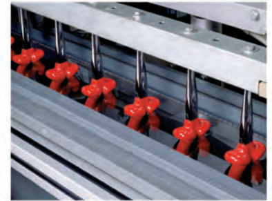
Testing of the electric insulation resistance
